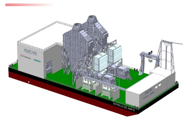
Estrella Del Mar III is a floating power plant capable of delivering a nominal net power output of approx. 145.5MW at design condition to the shore power system via two export feeders at 69kV voltage level.
