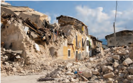
Natural Disasters; Wildfires; Landslides; CBRE incidents
